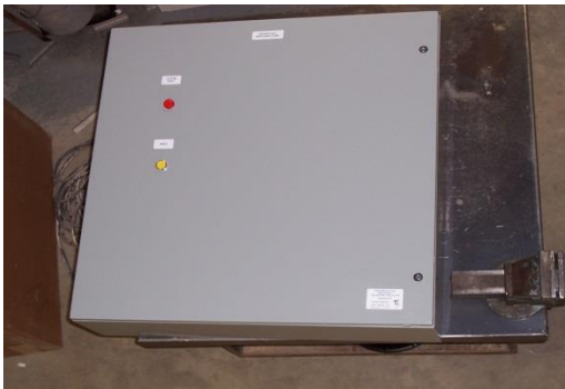
Cover of Typical Large GFI Panel
